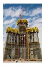
The WOLFF 355 B luffers are raised step by step with the building by means of an internal climbing procedure. One luffer will be replaced several times and will reach a final hook height of around 800 meters.
