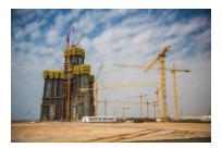
Working on behalf of the Saudi Arabian construction and real estate company, Saudi Bin Ladin Group, Roots Group is currently using thirteen WOLFF cranes for the construction of the Jeddah Tower, which will be the tallest building in the world at over 1,000 meters above sea level.
